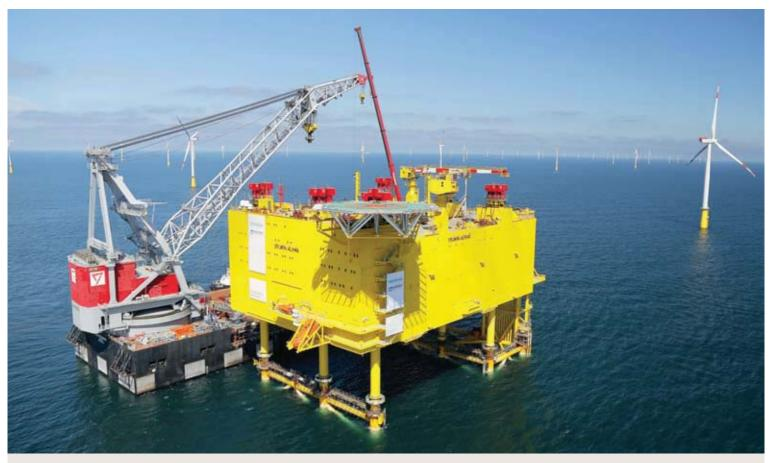
The SylWin alpha platform (864 MW) is the world's largest installed converter platform. It will transmit the energy produced by the three North Sea wind farms DanTysk, Butendiek and Sandbar ashore.
